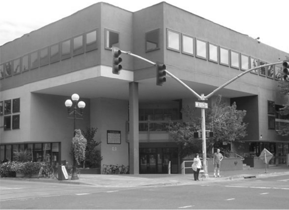
Figure 4. The Atrium Building, the site of the Lane Independent Living Alliance. Photo Source: LILAOregon.org.
